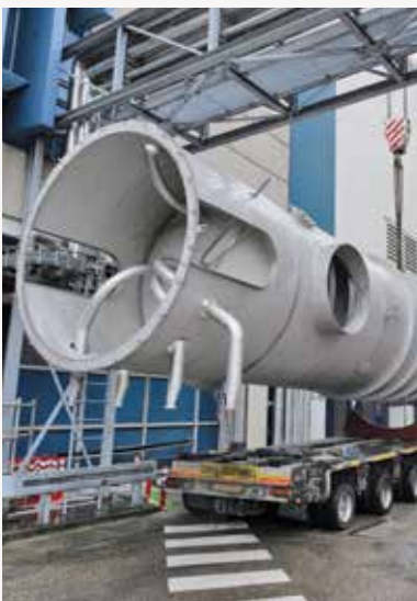
Installing new condensers in Leeuwarden (Netherlands)
